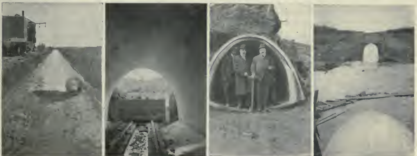
Various construction views of aqueduct—Greater Winnipeg water supply.
